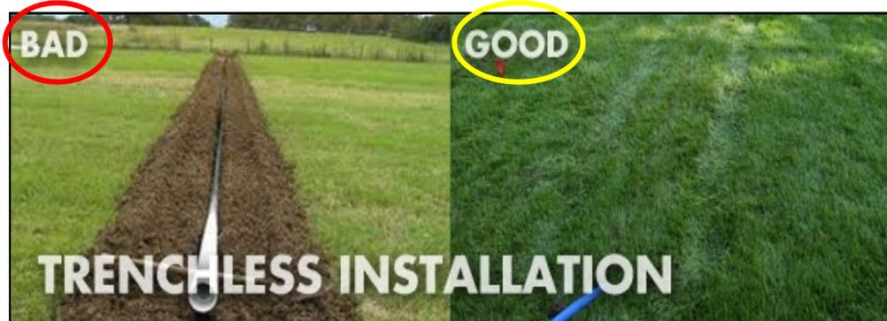
The bad vs the good. The photo on the left is NOT the way we install systems. This method requires extra steps after installation to repair the lawn. The photo on the right shows what it looks like when we install systems. Using a vibratory plow, we pull the pipe underground without disturbing the surface of your lawn.
